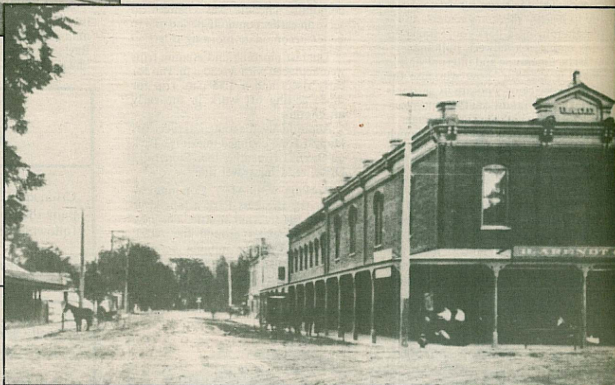
The 450 Main Street Building, 1900, now under renovation.
