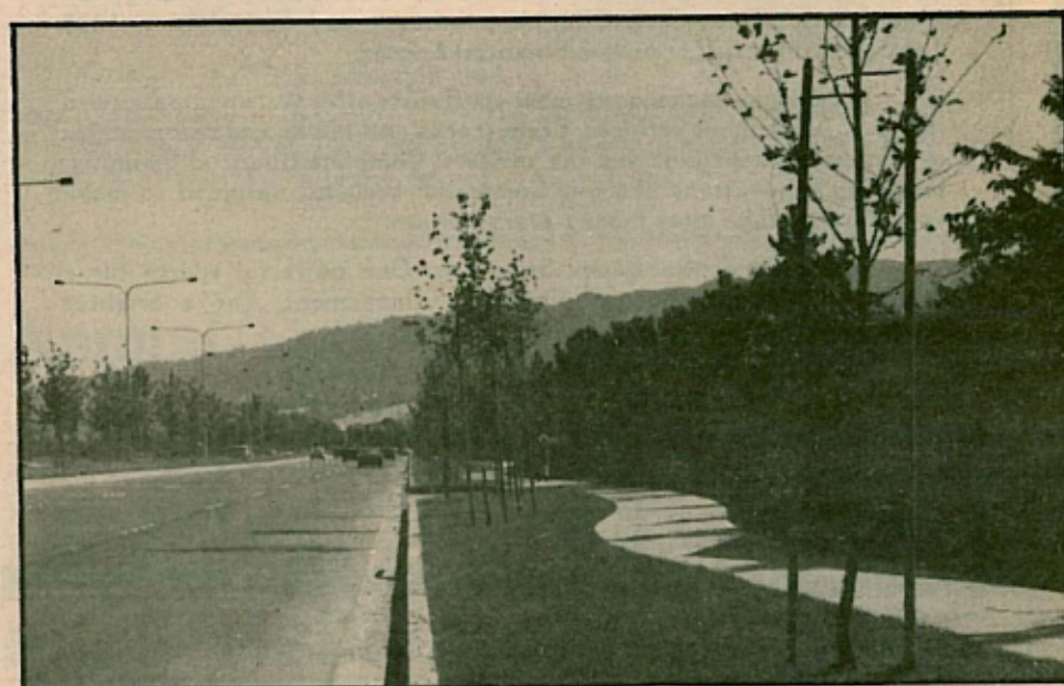
Sidewalks and street lights are part of city improvements from development in North Pleasanton.
