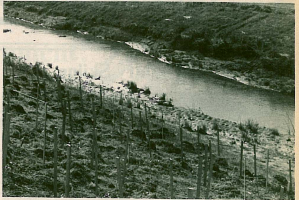
Wooden stakes mark where newly-planted shrubs and grasses are helping re-vegetate the banks of Tassajara Creek.
