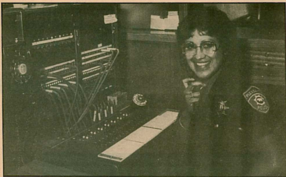
Angela Calya of City Hall works at the old switchboard which will soon be replaced by a new phone system.
